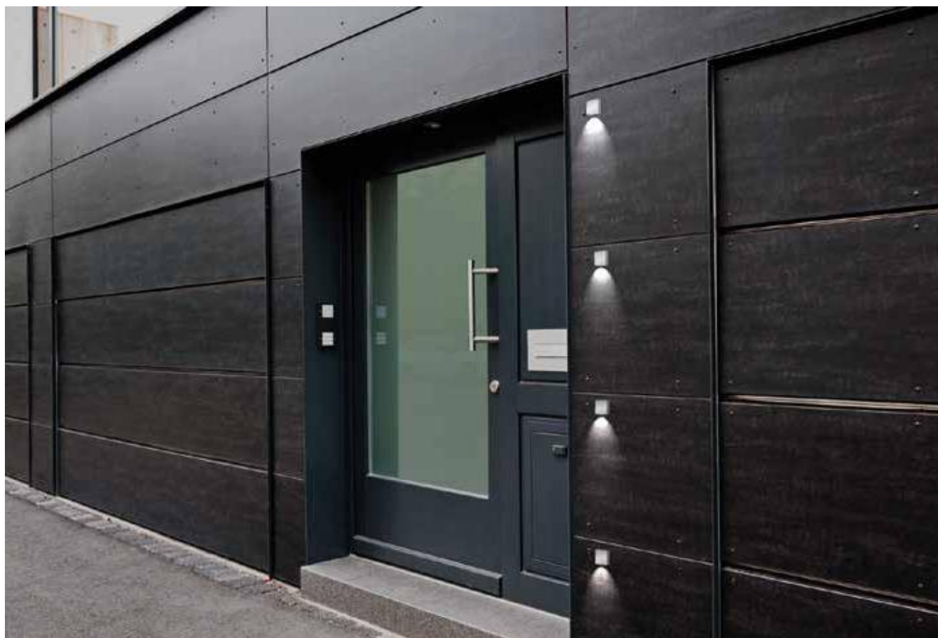
EXTERIOR LIGHTING WALL LIGHT - Recessed
