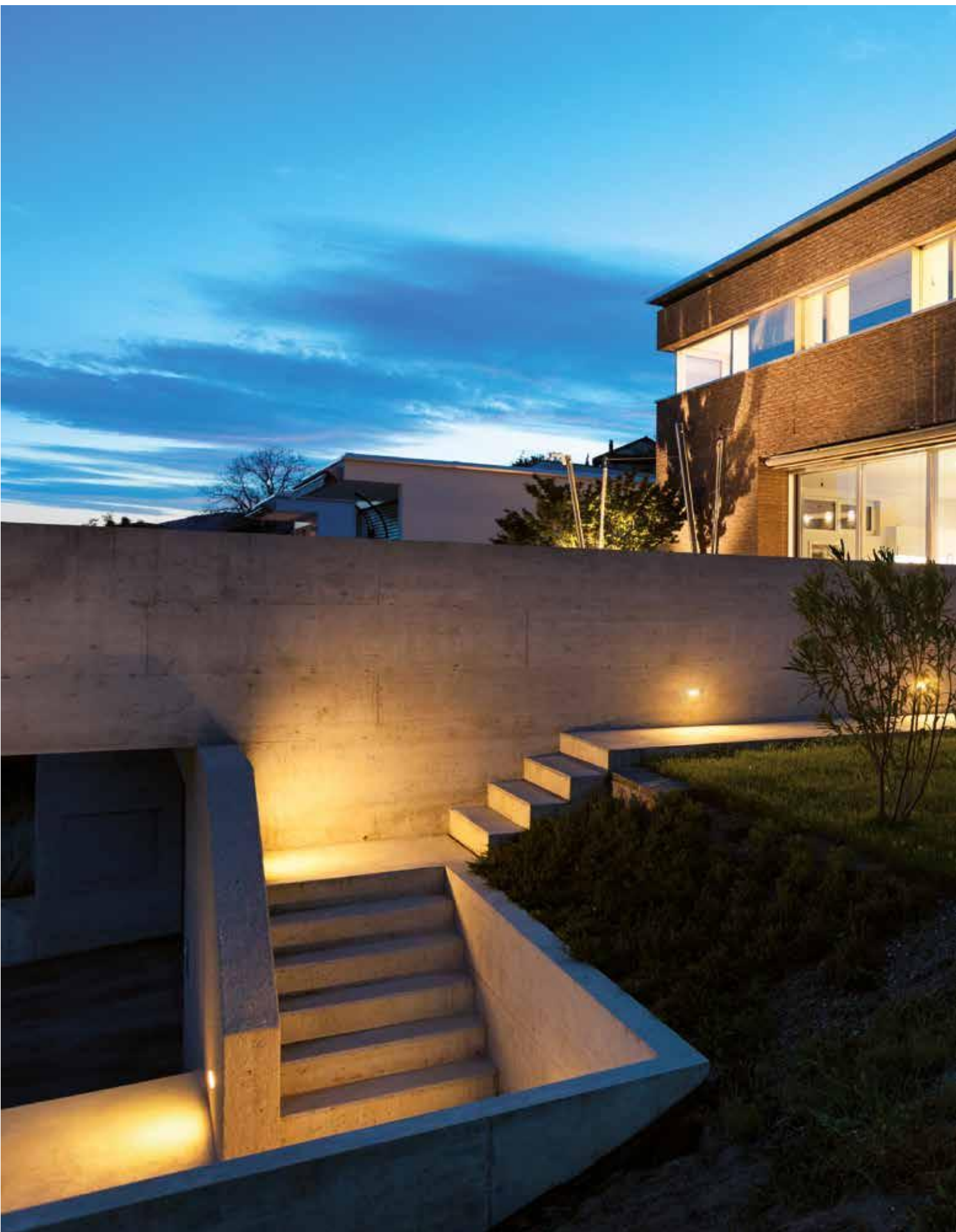
EXTERIOR LIGHTING WALL LIGHT - Recessed
